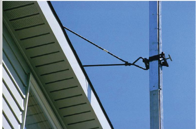
A Pump Jack scaffold's triangular bracing.
